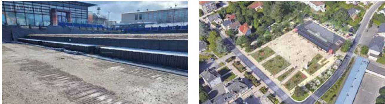
2,300M 3 - SAINT JEAN DE BRAYE As the city had already been impacted by flooding in 2018, the city authorities chose to redevelop the city centre and to construct a rainwater storage basin under the city esplanade, prior to proceeding with town square greening works to benefit inhabitants; this is an example of integrating such structures into the urban landscape.
