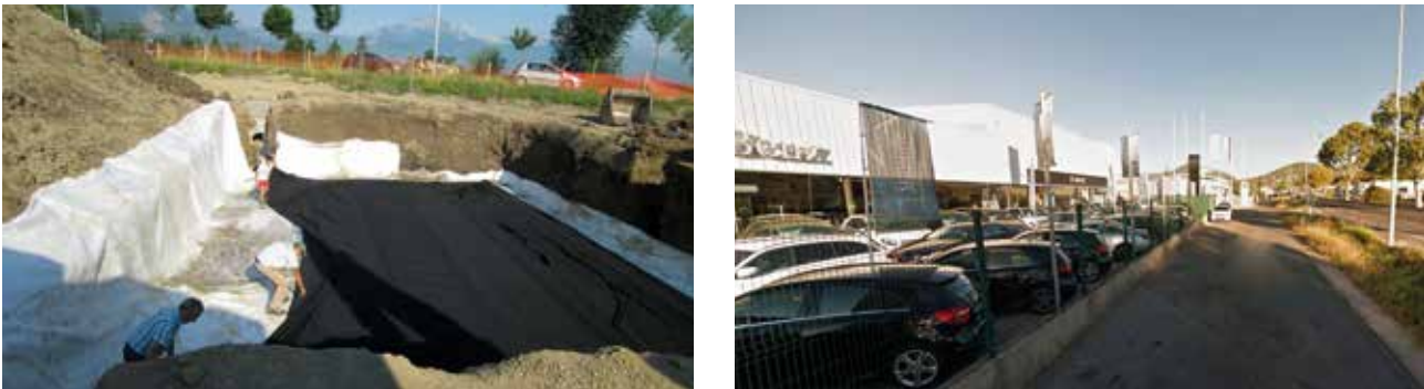
180M 3 - LA GARDE Waterproof basin located near La Garde Mercedes dealership (Var department), for stormwater runoff storage.
