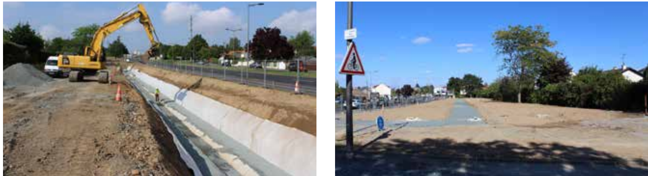
2,500M 3 - CHOLET Two underground basins, located on either side of an existing collector, were built near a busy road to address flooding issues in this area.
